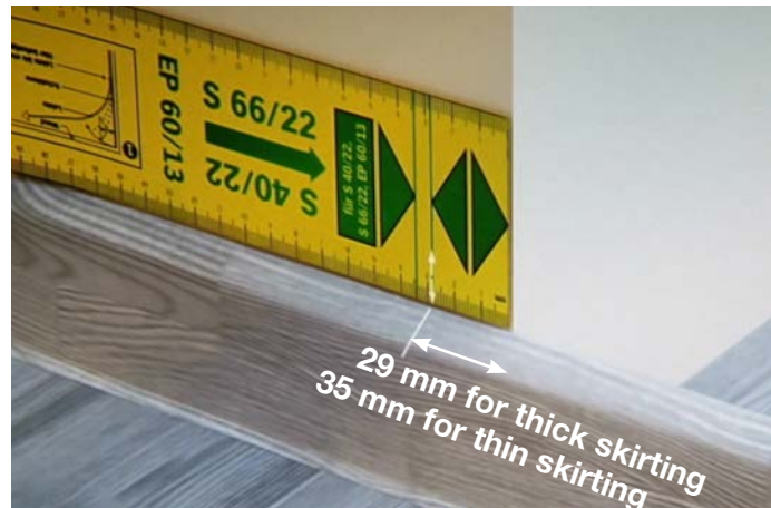
Mark the solidcore skirting accordingly
