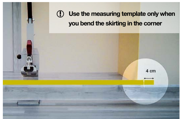
Mark the solidcore skirting accordingly
