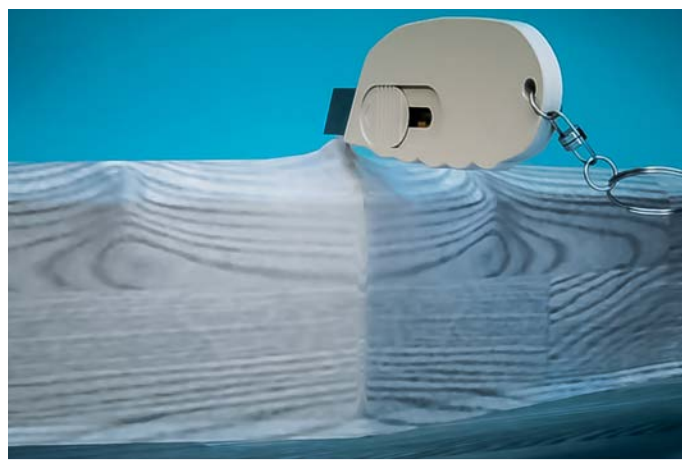
Cut out the bowing on the upper flexible lip
