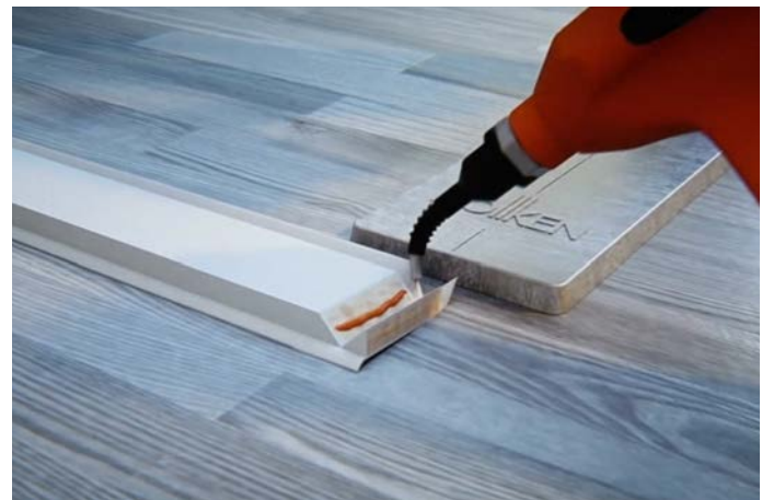
Use Döllken hot melt to fix the end caps
